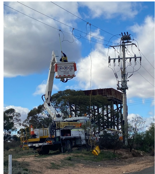
Specialist electrical contractors completed all high voltage/low voltage electrical checks at the Buronga and Coomealla pump stations.
