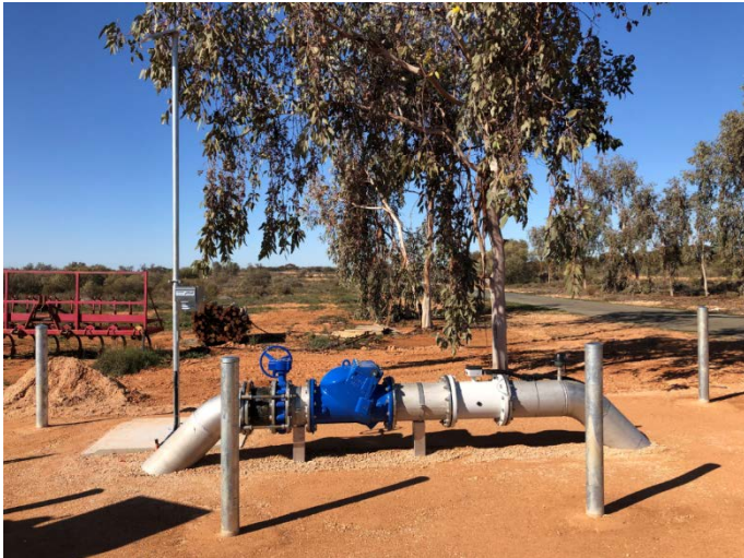
The first 300mm meter & telemetry installation in Coomealla is complete.
