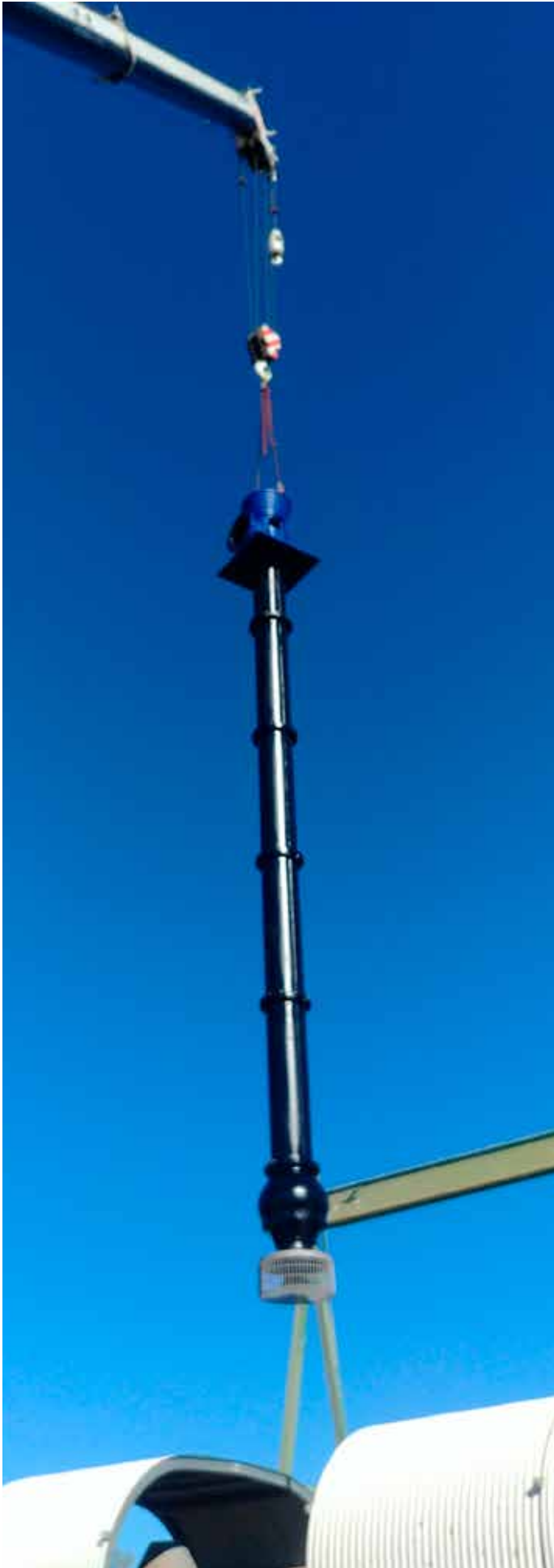
The second new KSB pump being installed at the Coomealla pump station
