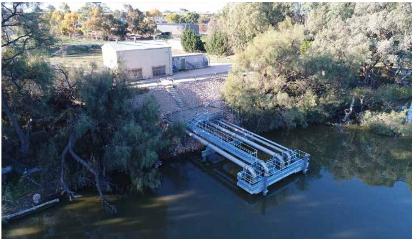
▲ Buronga pump station with its new suction jetty walkway and upgraded stair access.
