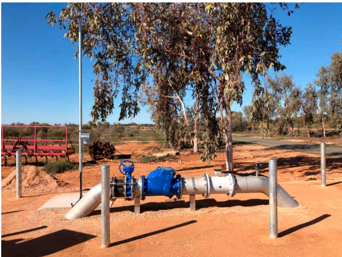
▲ The first new 300mm meter and telemetry installation in Coomealla
