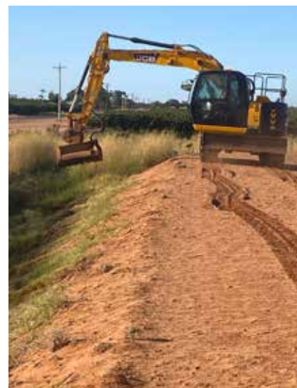
▼ Enhanced maintenance of surface drains with dedicated contractors
