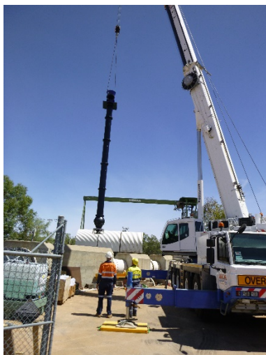
The third new KSB pump being installed at the Coomealla pump station in March.
