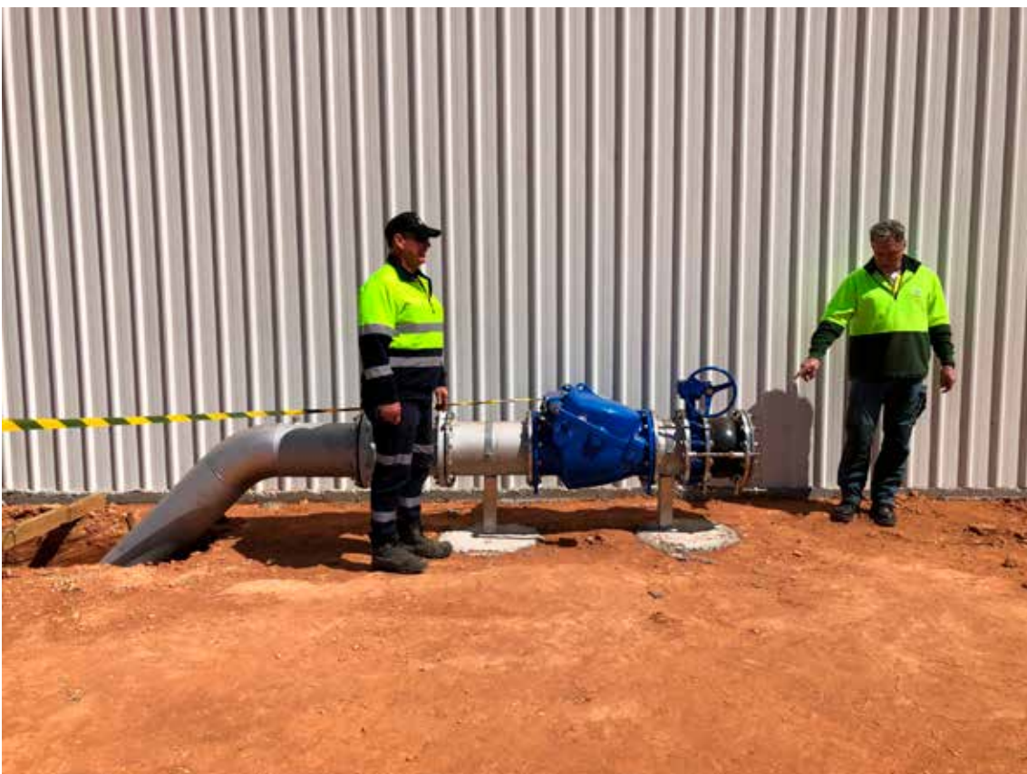
◀ The second 300mm outlet in Coomealla ready for customer connection.
