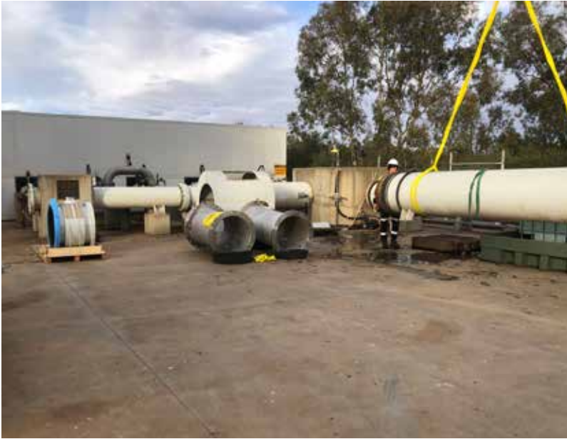
▲ New Curlwaa main mag meter being installed.
