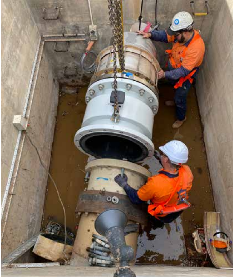
▲ New Buronga pump station mag meter being installed.
