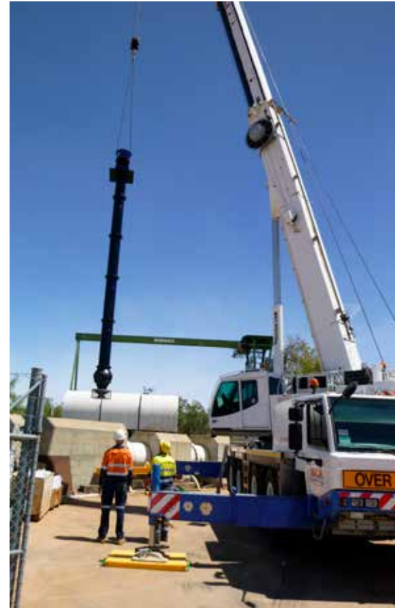
▼ The third new KSB pump being installed at the Coomealla pump station.
