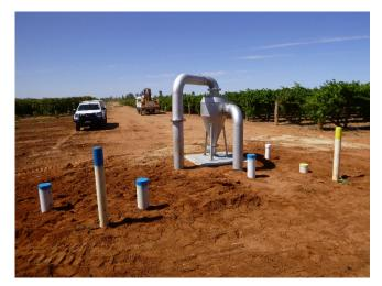
Recently installed cyclonic filter will be trialled to assess the effectiveness of removing shells.
