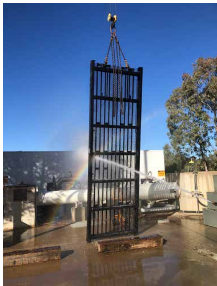
> TOP: Cyclone filter trial to assess effectiveness of shell removal prior to customer outlets – installed near Bernarra Road, Coomealla > LEFT: Curlwaa pump station trash rack cleaning > RIGHT: Extensive surface drain maintenance at Syphon and Hollands Lake Roads, Coomealla
