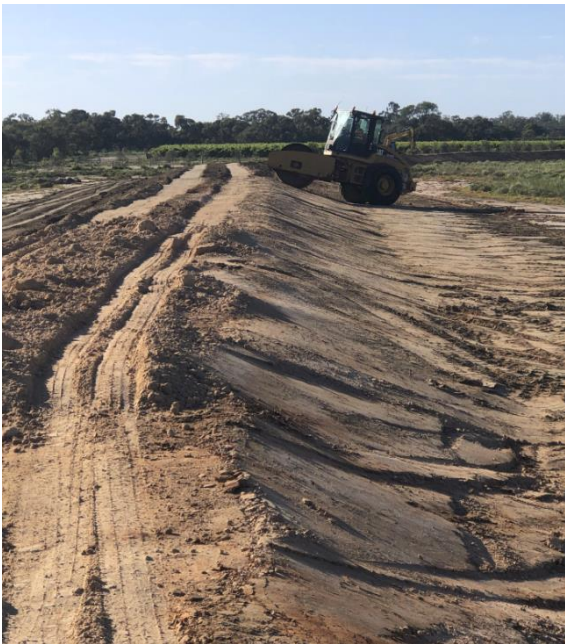
Strengthening the Curlwaa levee began in October 2022.
