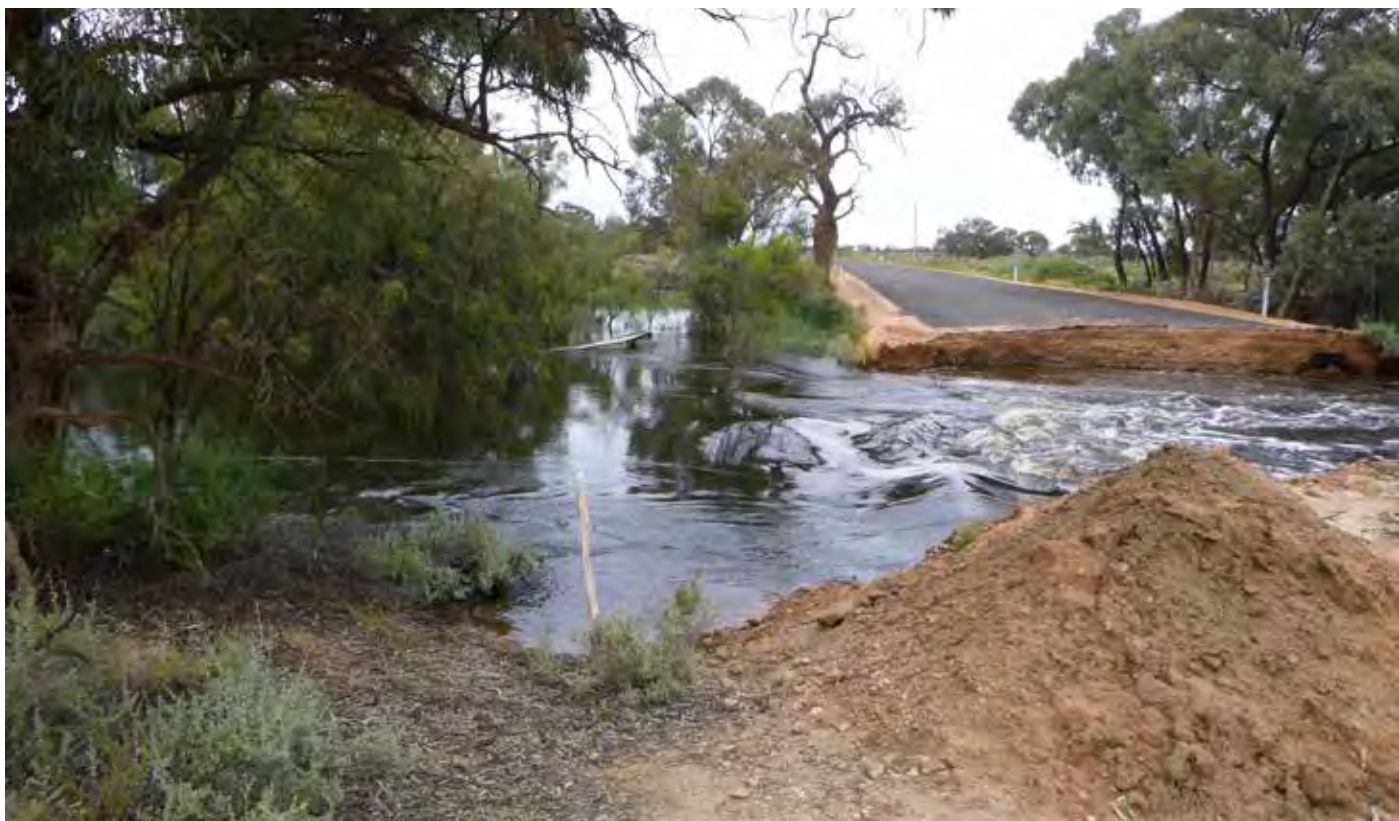
> TOP: Wentworth Shire Council cut through Old Wentworth Road to alleviate the build-up of pressure on the Curlwaa levee from Tuckers Creek. Water was then directed naturally into Fletchers Lake.
