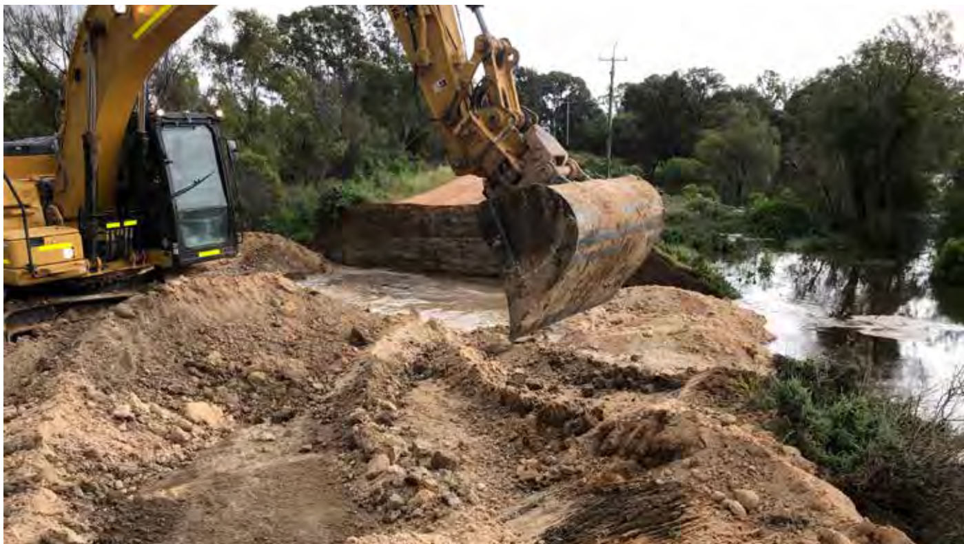
> TOP: Repairing the Curlwaa levee breach
