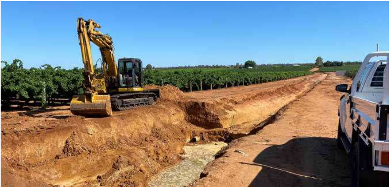
> Surface and deep drain storm repairs: Coomealla
