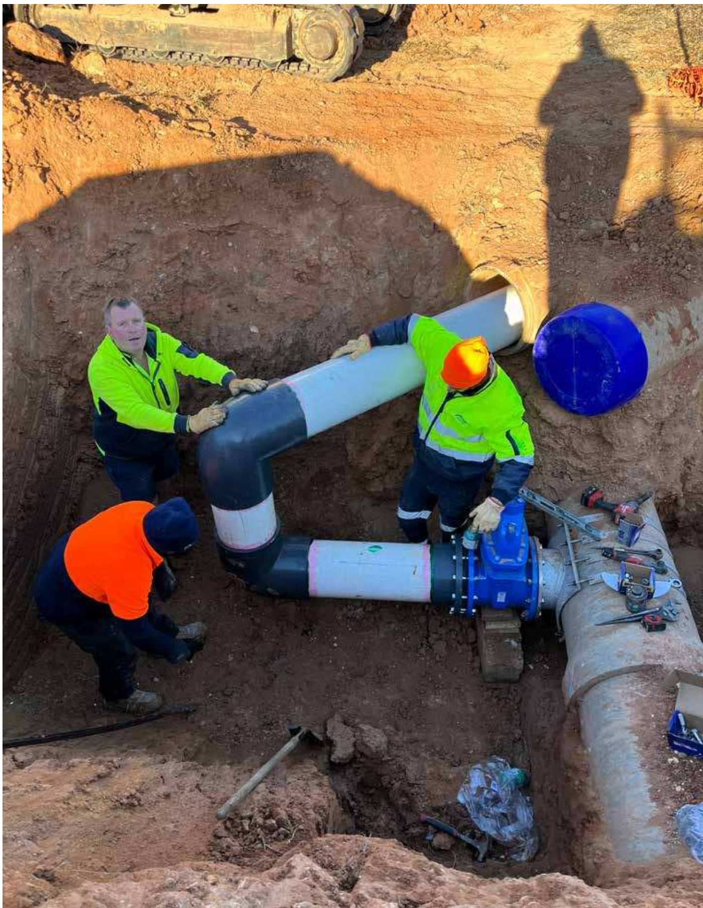
> Northern end of Keenans Drive Coomealla: New scour install
