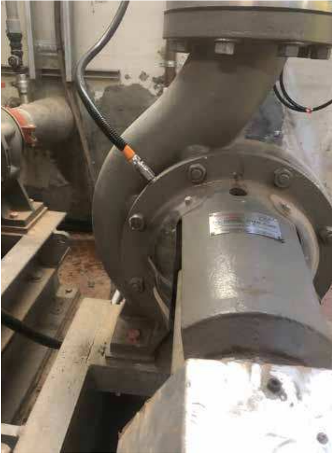
> Buronga Pump D vibration sensor location (vibration monitoring system completed)
