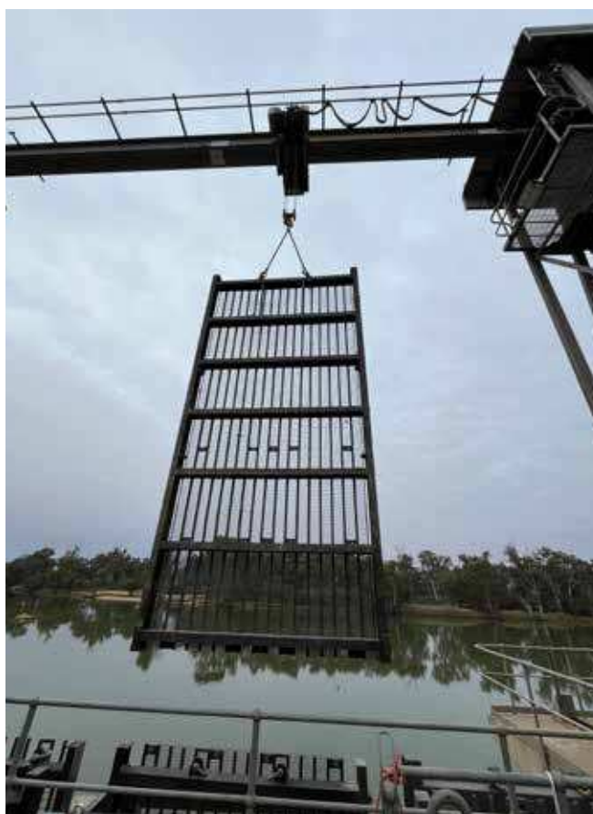
> Curlwaa trash rack removal for cleaning
