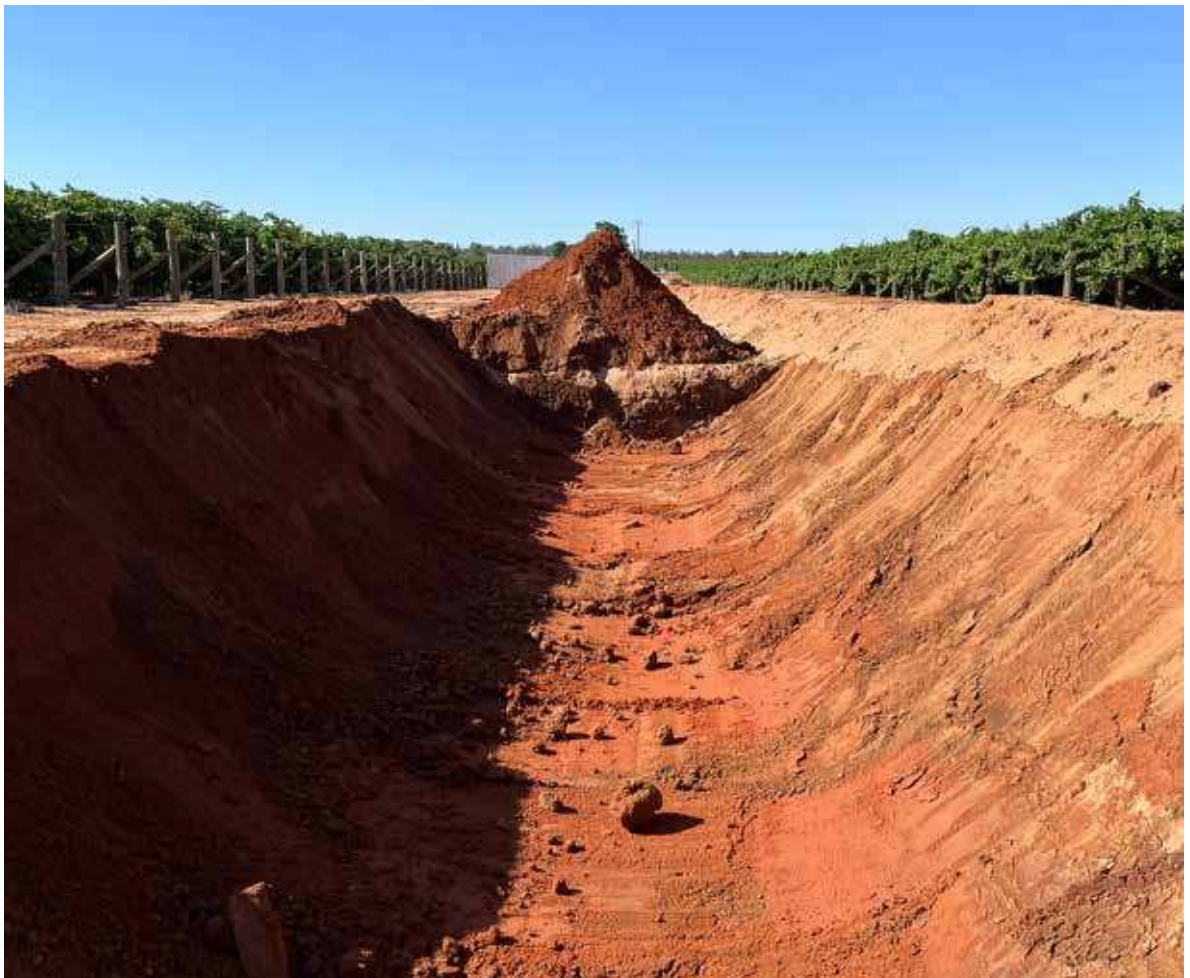
> Coomealla: 27 Truck loads of silt removed
