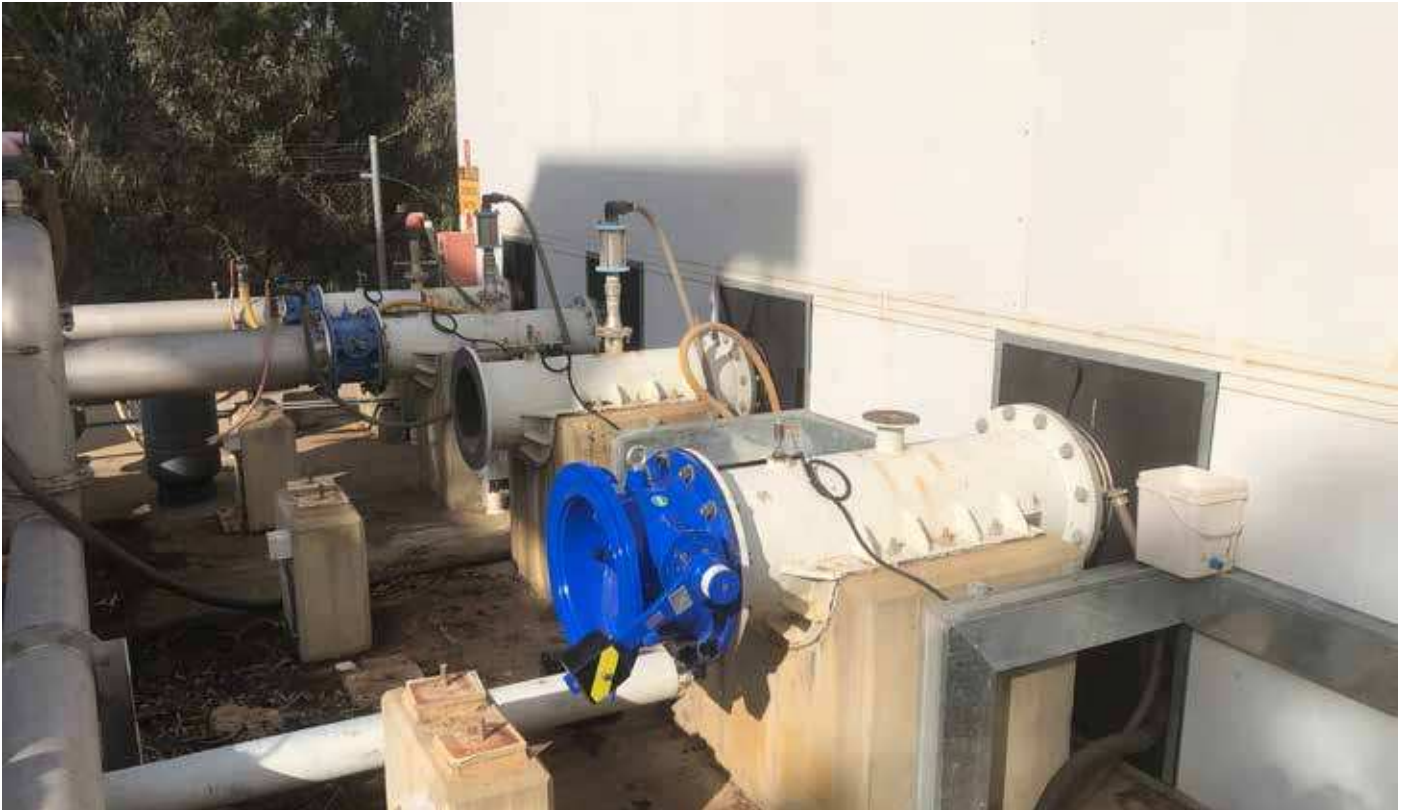
> New check valves for Curlwaa Pump C&D
