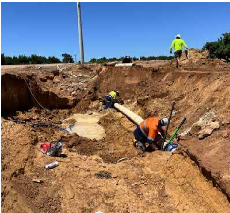
> Surface and deep drain storm repairs: Coomealla
