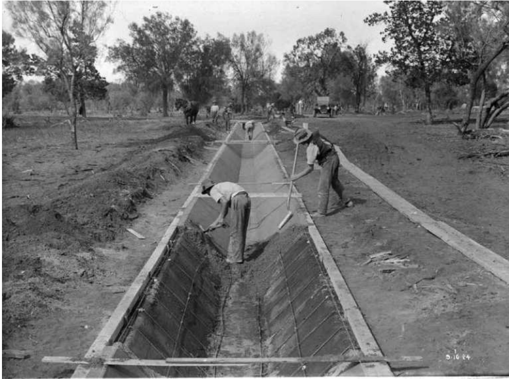
> ABOVE: Construction of channels, 1924 > BELOW: Construction of the rising main, 1924
