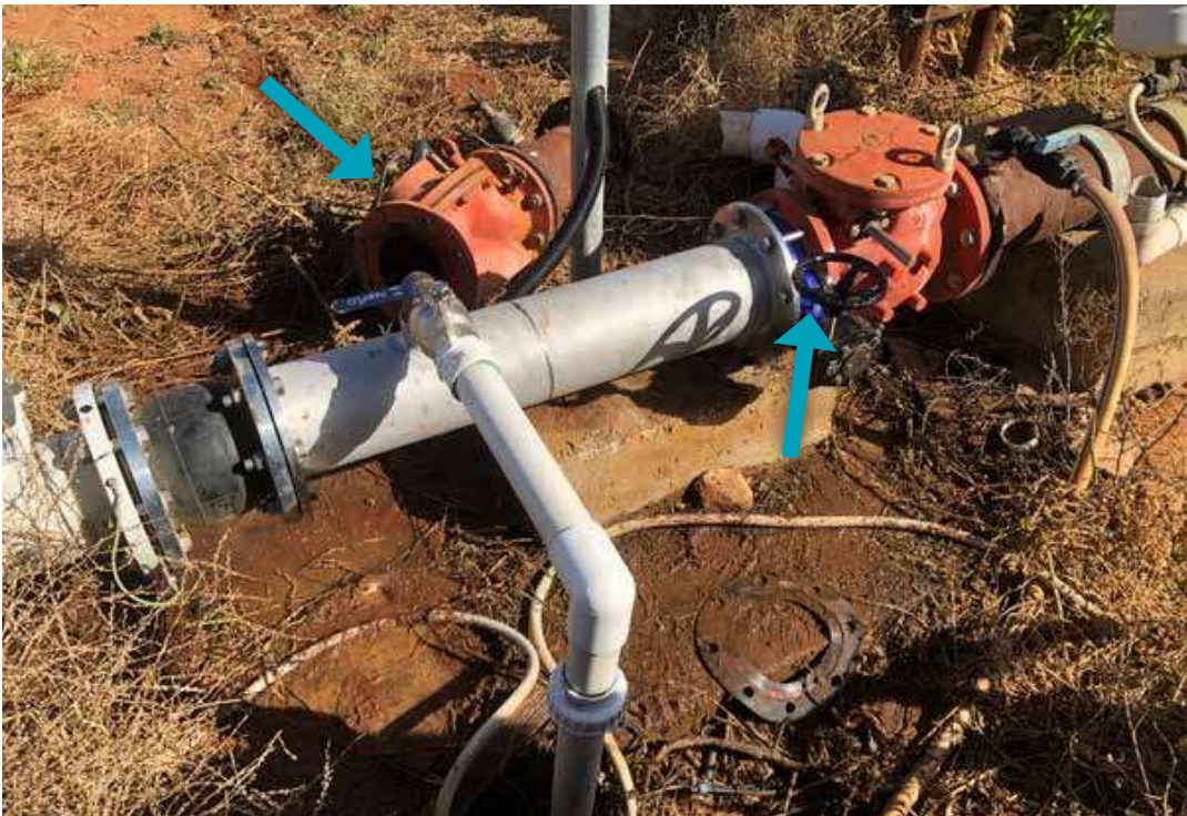
> Buronga Pump D vibration sensor location (vibration monitoring system completed)
