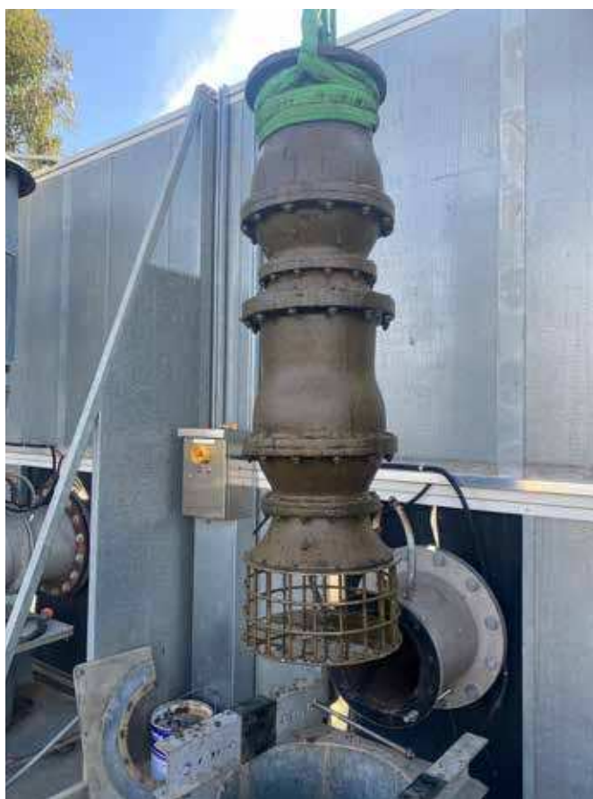
> Curlwaa pump D removal for service overhaul
