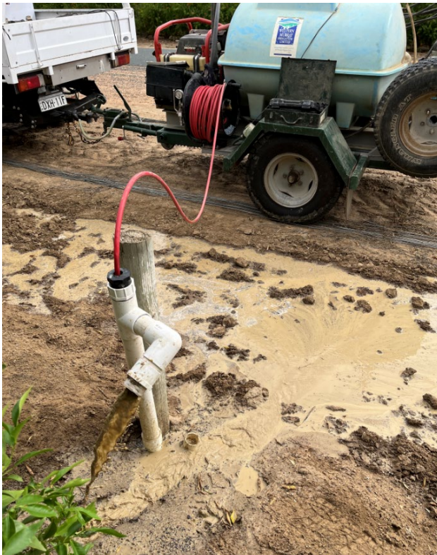
Example of piezometer desilting in progress. This piezometer was previously 'dry', it is now 2M deeper. Will be checked for reading in 2 weeks.
