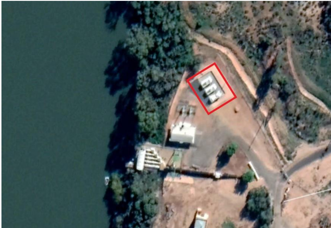
Figure 2: Location of Generators and Diesel Fuel Tank
