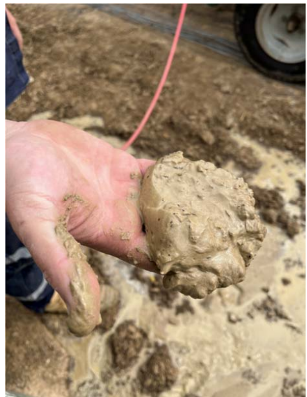
Example of piezometer desilting in progress. This piezometer was previously 'dry', it is now 2M deeper and reading correctly.
