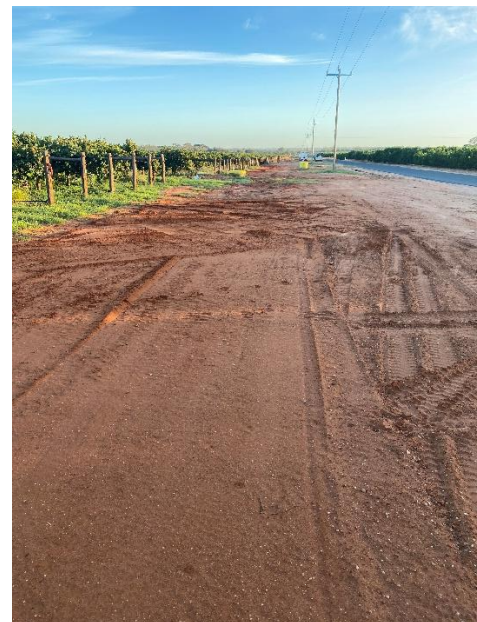
Completed repairs 31 March 2026
