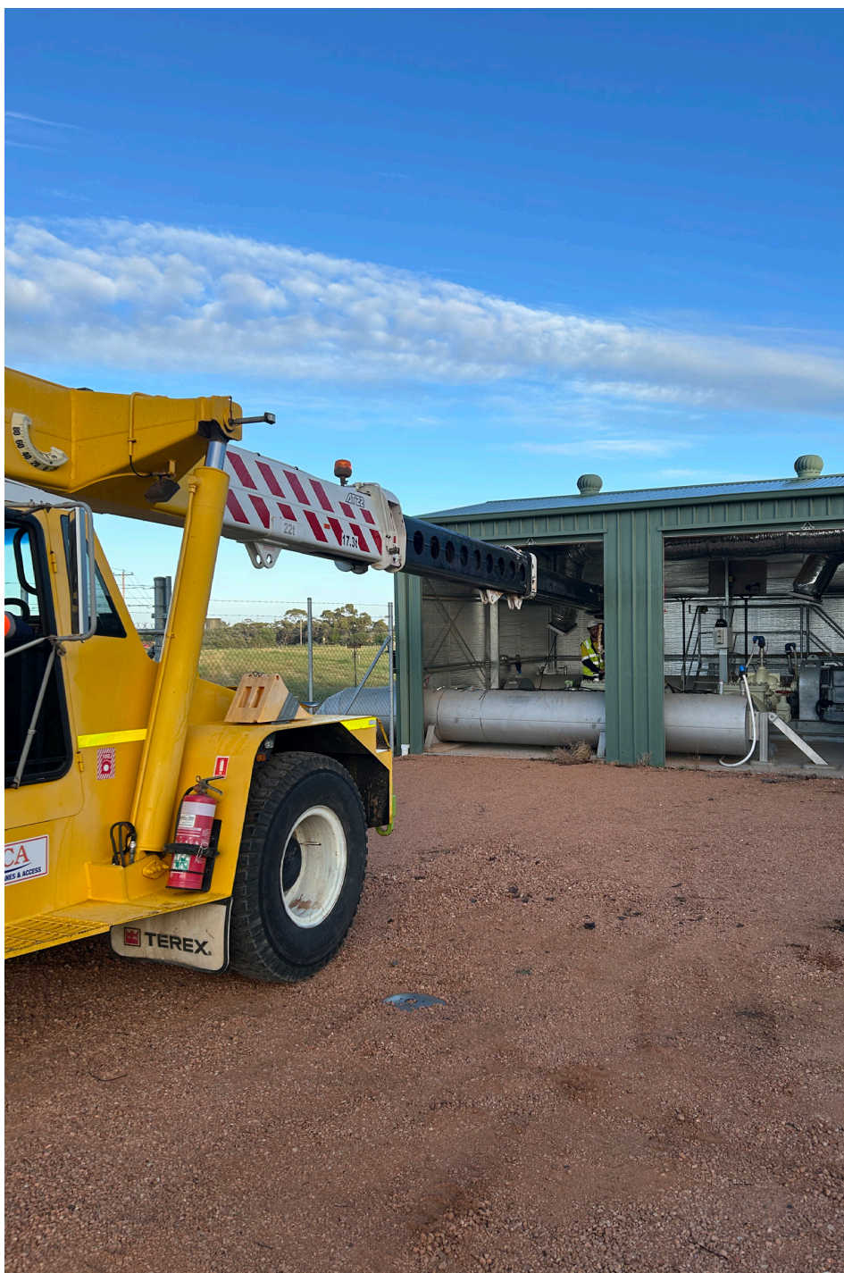
> LEFT: Coomealla Relift Station pump B being removed for overhaul
