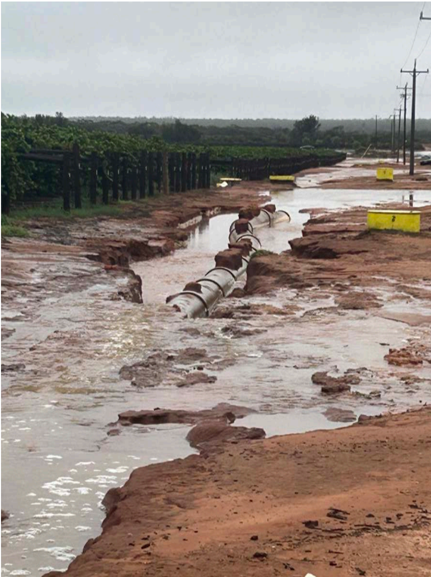
> ABOVE LEFT: Coomealla Hollands Lake sub surface drain damaged by the record rainfall: 2 March 2026
