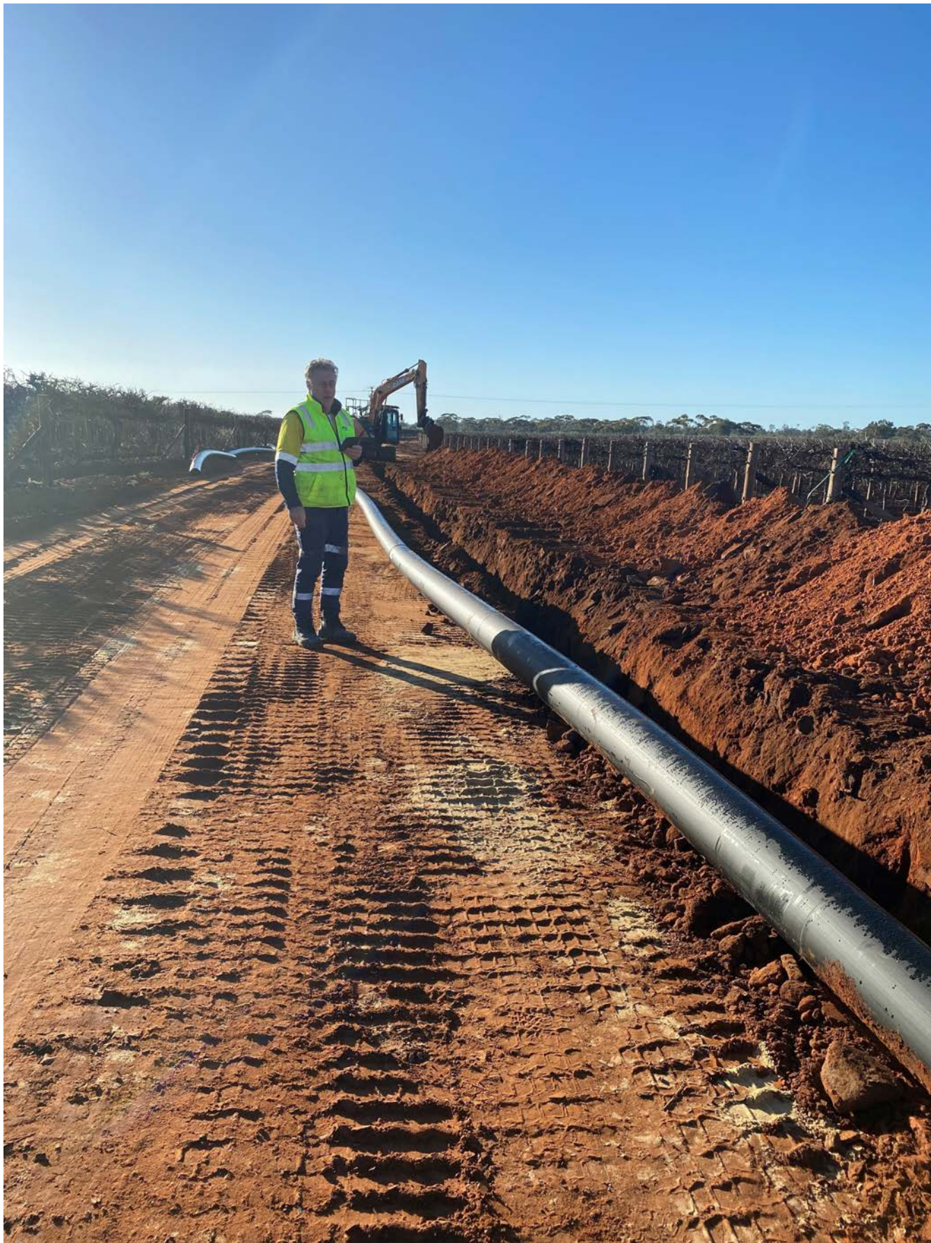
> ABOVE: Commenced Coomealla Lateral 7 pipeline upgrade
