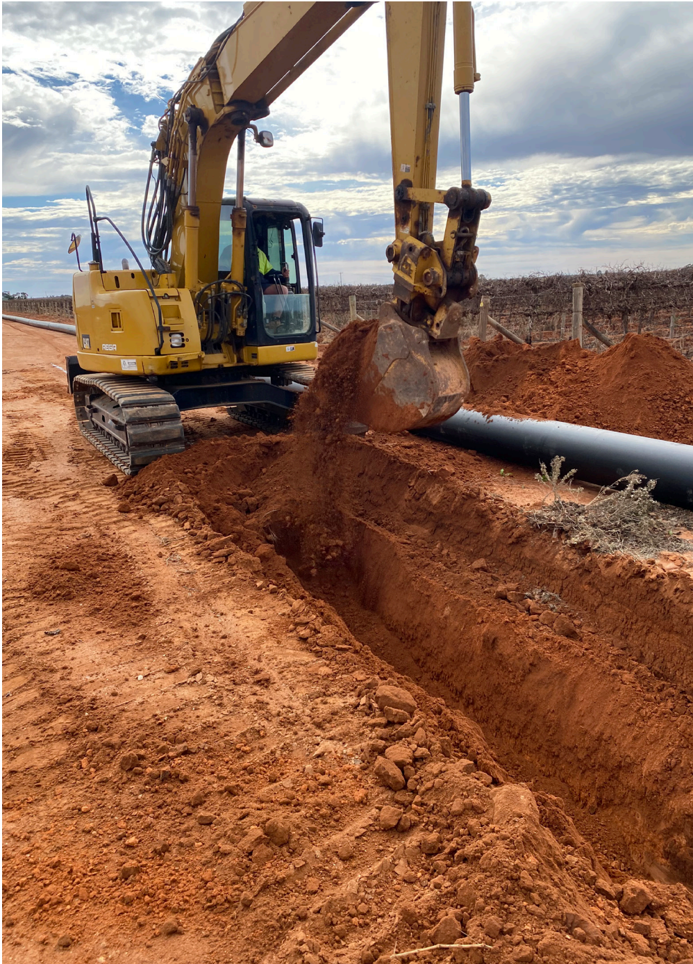
Completed and commissioned Coomealla Lateral 30 pipeline upgrade
